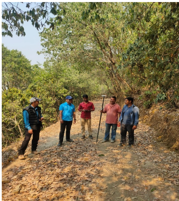
Observation and Survey of Access Road to Siddhapark
